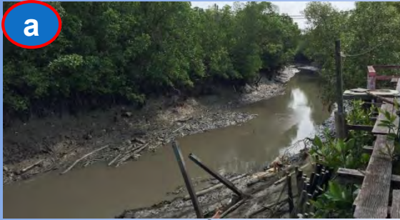
Inner section of the waterways
